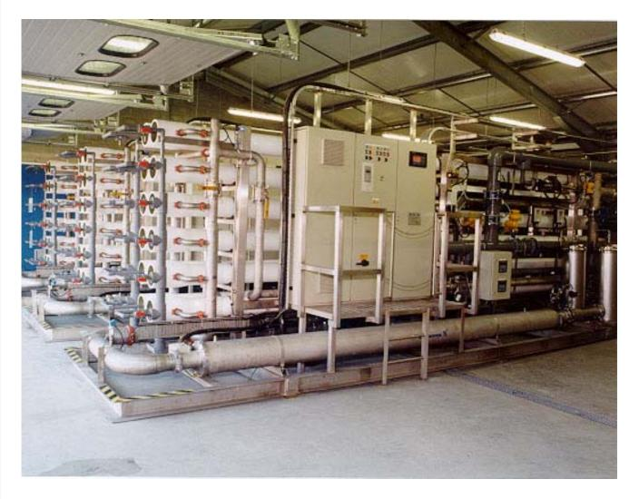
Reverse osmosis provides a primary purification stage, using a semi-permeable membrane to reduce ions and other contaminants, up to 99%. Aqueous solutions will permeate through a semi-permeable membrane to equilibrate the ionic concentration on either side of the membrane. This process is known as osmosis, in reverse osmosis pressure is applied to the concentrated solution to drive water through the membrane and produce permeate with a lower concentration of ions than the feed water.
